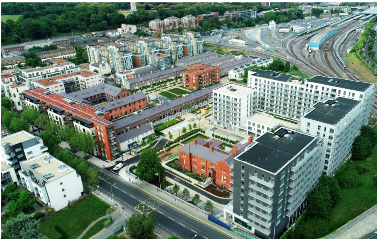
Figure 14.4.2.7.7 Aerial view of the former Clancy Barracks (RPS 1851 / Multiple NIAH entries) now reused to form the Clancy Quay development.
