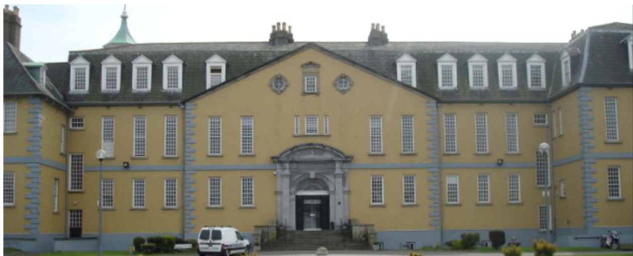
Figure 14.4.2.7.12 Dr Steevens's Hospital, St. John's Road West, Dublin 8
