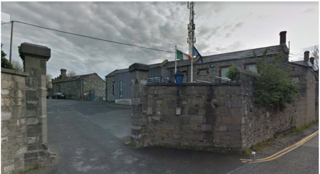
Figure 14.4.2.7.4 Kilmainham Garda Station Complex, Kilmainham Lane (RPS 4256 / NIAH 50080065 / 50080066)
