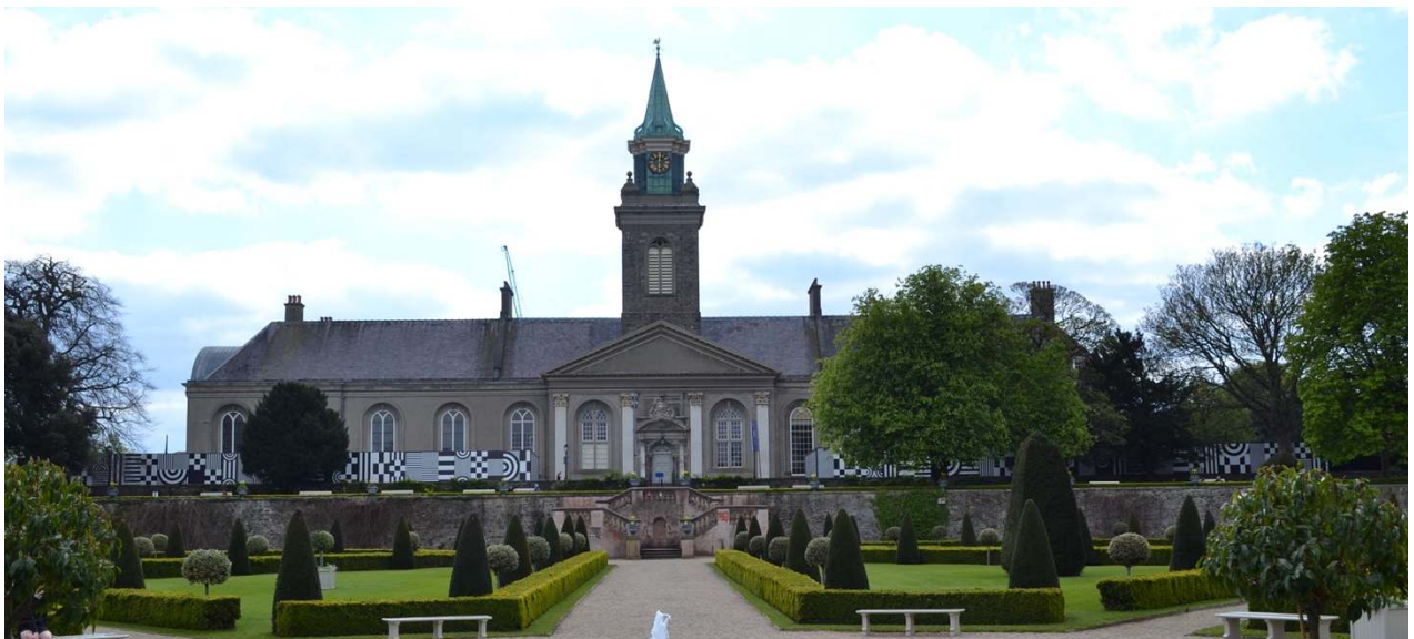
Figure 14.4.2.7.1 The principal (north) elevation of the RHK (RPS 5244 / NIAH 50080072).
