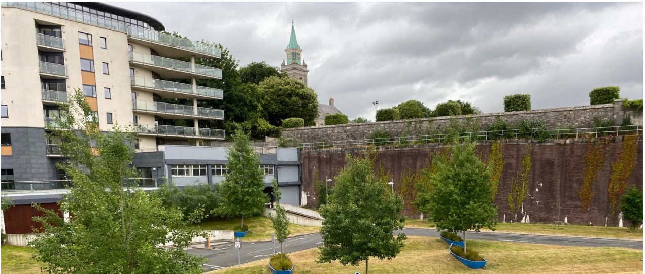
Figure 14.4.2.2 View towards the boundary wall of the RHK gardens from the decked area of the HSQ site above the car park.
